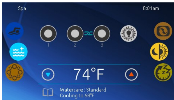
Figure 1: Main screen with pumps off
